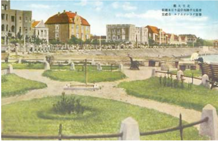
At upper right, the three buildings of the Grand.
